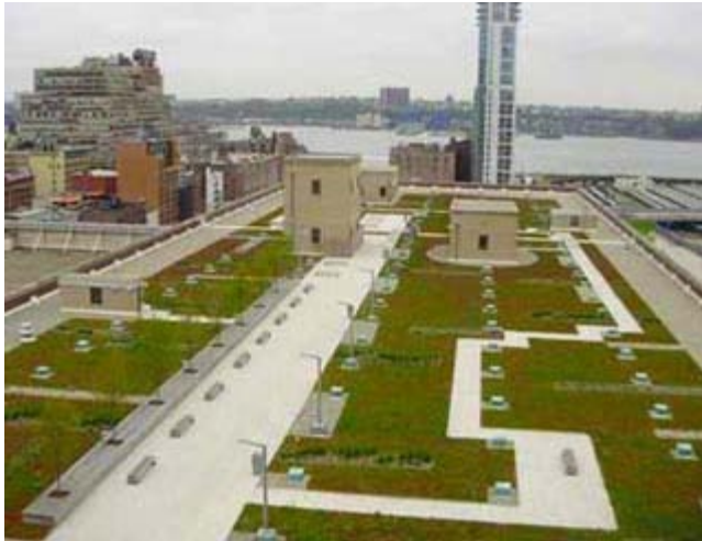
The New York City skyline provides a scenic backdrop for the U.S. Postal Service's green roof.
